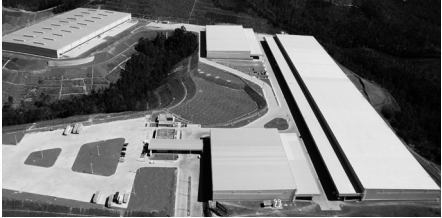
DP Cajamar Galpões Warehouses : 89.000 m²
