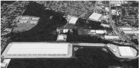
DP Manaus I Galpões Warehouses : 105.000 m²
