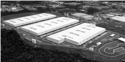
DP Manaus III Galpões Warehouses :133.000 m²
