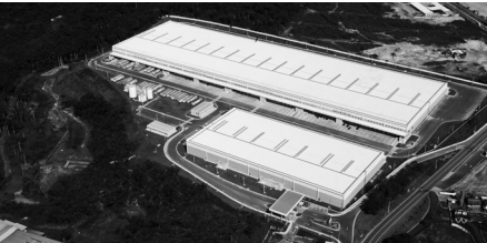
DP Manaus II Galpões Warehouses : 69.000 m²
