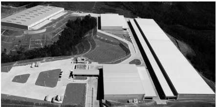
DP Cajamar Galpões Warehouses : 89.000 m²
