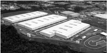
DP Manaus III Galpões Warehouses :133.000 m²
